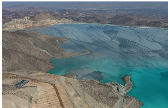
Figure 6(c): Image of mine tailing pond
